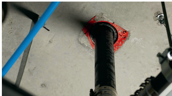
Fig. 15: Device flange should be secured to the top surface as per listed system Hilti CFS-DID
