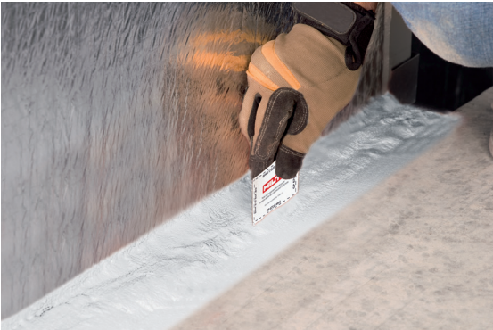
Fig. 34: Correct depth of sealant, Hilti CFS-SP SIL
