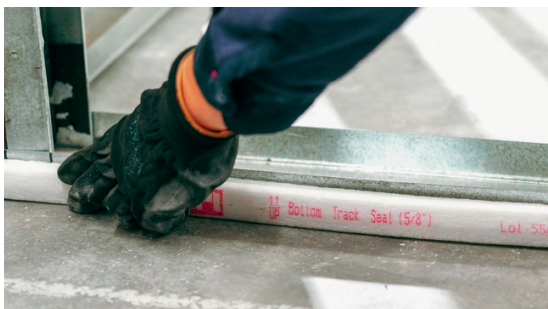
Fig. 28: Bottom track seal installed on floor runner
