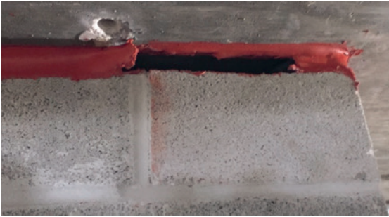
Fig. 30: Gap in application
