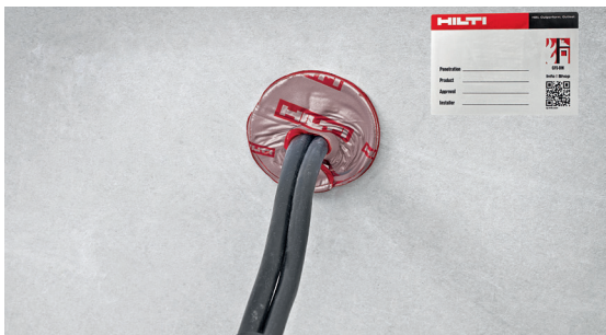
Fig. 14: Fire protection cable disc, Hilti CFS-D used for sealing a cable bundle of size < 1 in. Watch the video
