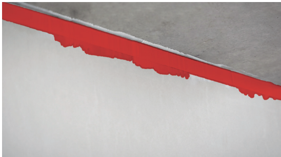
Fig. 24: fire protection sealant applied to the top-of-wall joint
