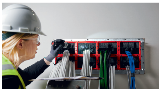
Fig. 13: Group of modular sleeves with gang plate for sealing multiple cable bundles of different sizes Hilti CFS-MSL GPA. Watch the video
