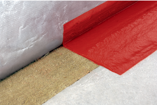
Fig. 33: Sealant Hilti CP-672, application in edge of slab assembly
