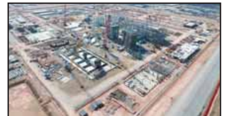
Petronas RAPID project, Pengerang, Johor
