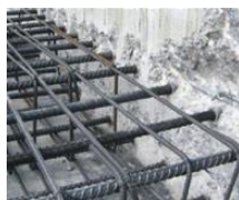
Slab to diaphragm wall
