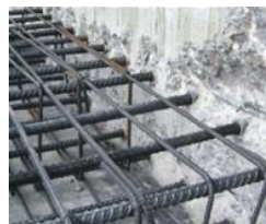
Slab to diaphragm wall
