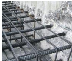
Slab to diaphragm wall
