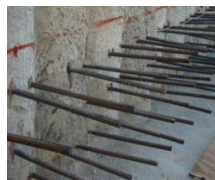
Slab to CBP wall
