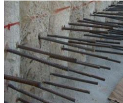
Slab to CBP wall
