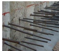
Slab to CBP wall
